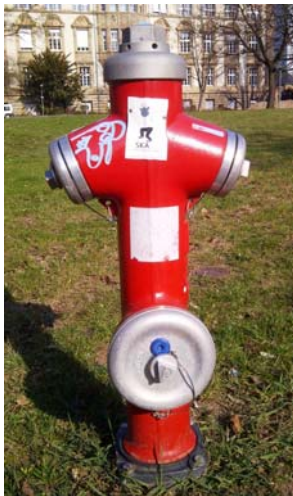
Fire Hydrant Maintenance
