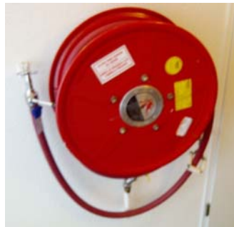
Fire Hose Inspection
