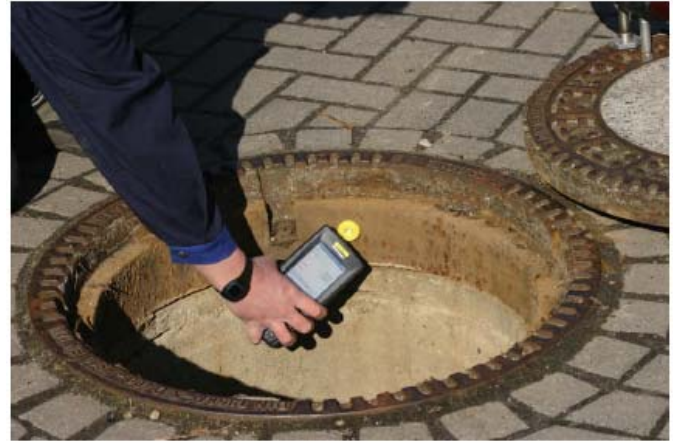
Manhole Maintenance & Repair
